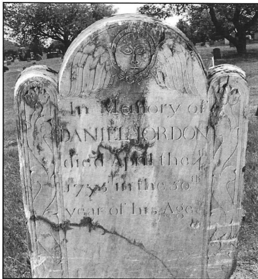
Fig. 23. Slate stone after conservation work.
