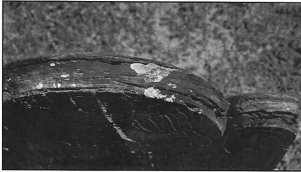
Fig. 22. Stone displays delaminating slate layers.
